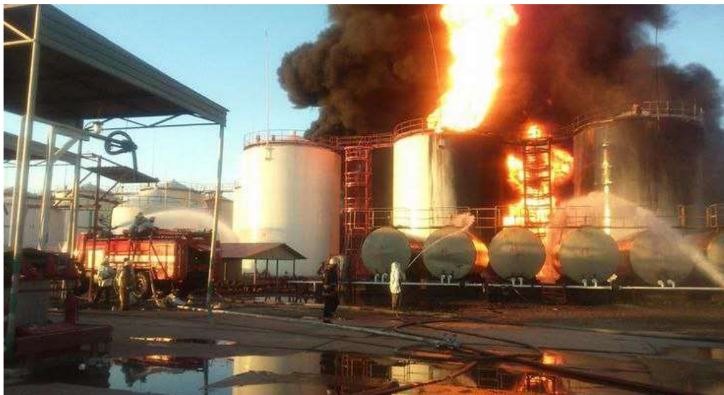
Fig. 3. Oil storage tanks explosions.
